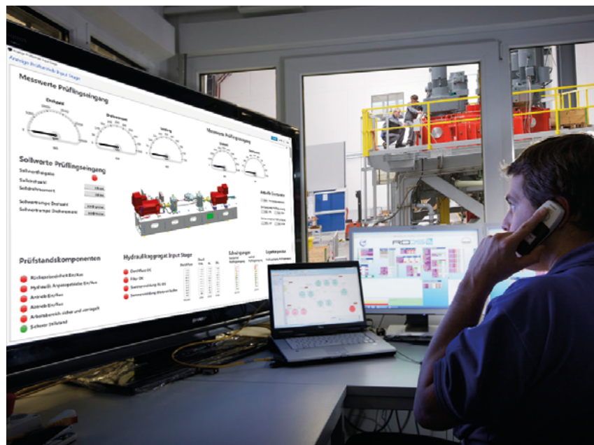
Example control room
